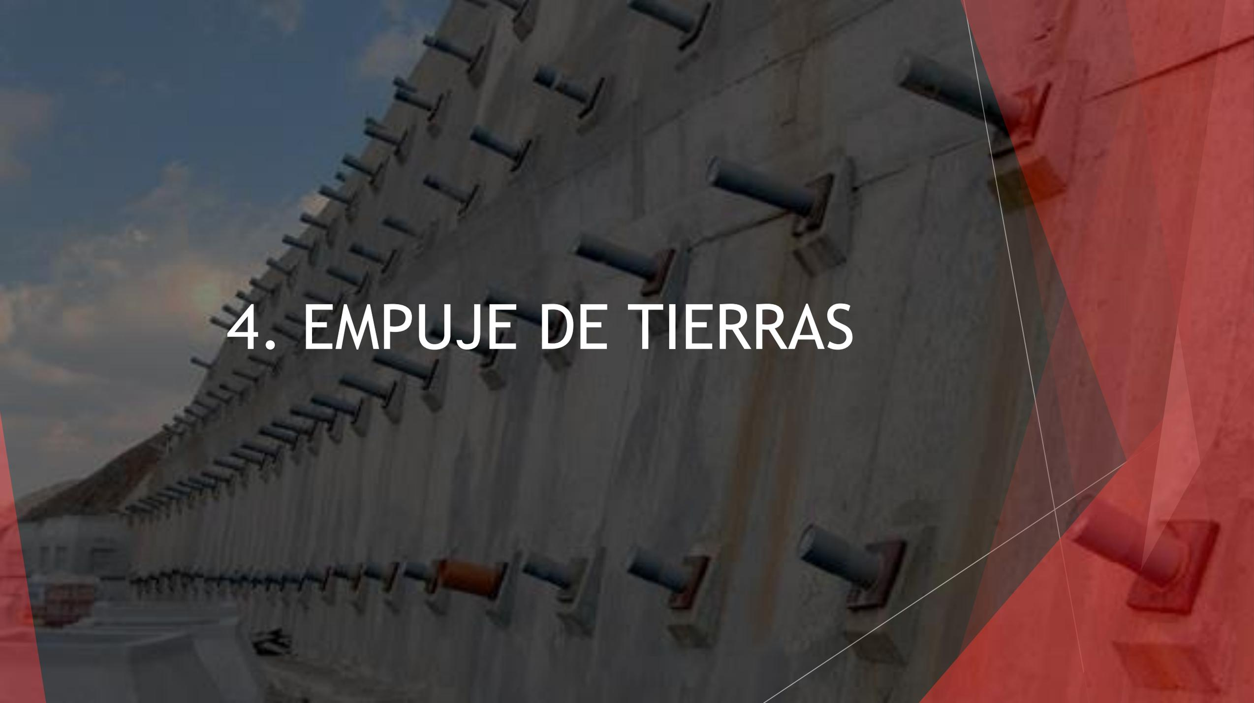
The background features a close-up, low-angle view of a retaining wall under construction. The wall is composed of grey concrete panels with numerous vertical steel soil nails protruding from them. The scene is set against a clear blue sky with a few wispy clouds. A large, semi-transparent red geometric shape, consisting of several overlapping triangles, is positioned on the right side of the image, partially obscuring the wall and sky. The overall lighting is bright, suggesting a sunny day.
